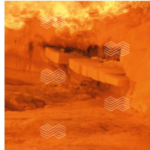
Установка DURITAL AZ58P / Installation of DURITAL AZ58P
