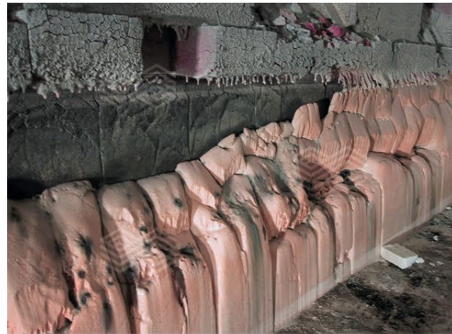
三年后DURITAL RK30NP外部贴砖 / DURITAL RK30NP overcoating tiles after three years
